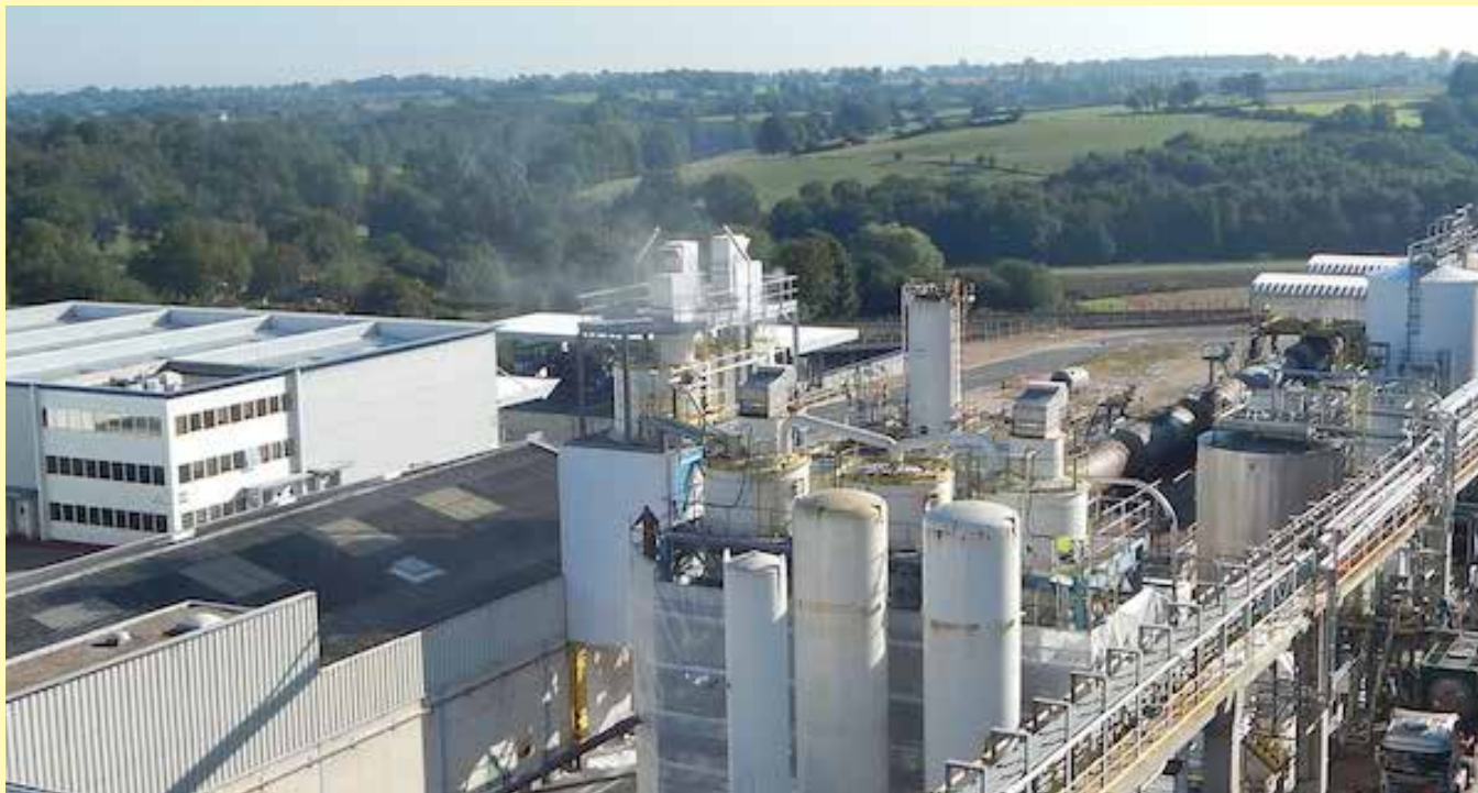
Adisseo's plant in Commentry, the birthplace of methionine production.
